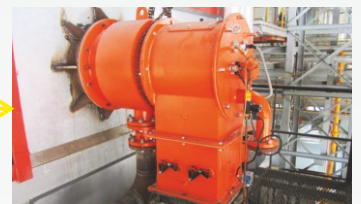
Biogas Burner for use in Boiler
